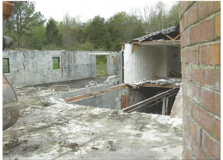
Demolition of the Castle was well underway in this photo.
