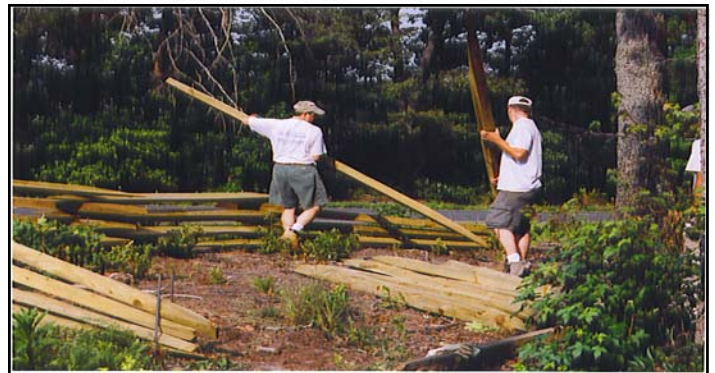
Mike Chapman and Eric Mink construct part of the worm fence
